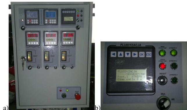
Fig. 3. System of controlling and recording operations of the thermal reclaimer a) General view, b) Control module of the fluidisation (bed mixing)
